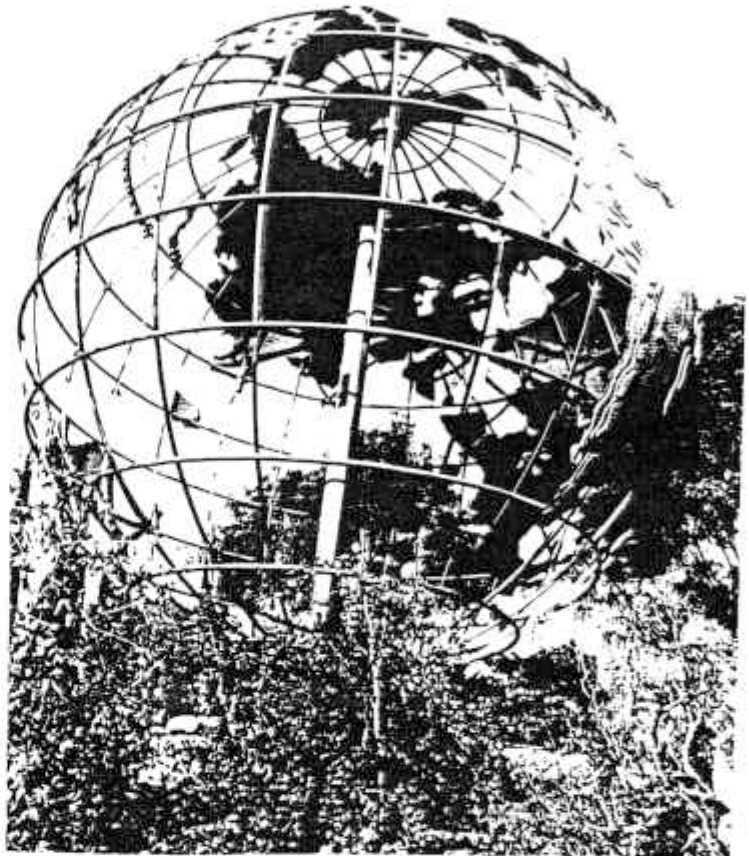
Neglected and unwanted, the "World", near St. George 's Episcopal Church on Avenida Carlotta, as it looked on February 1.
