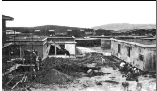
Paleontologists digging for fossils on Avenida Majorca in December, 1964. Building 207 is on the right.
