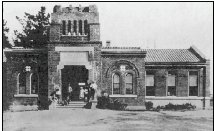
In 1913 El Toro's one-room school, built in 1891, was replaced by the red brick El Toro School, above. The one-room school was moved to El Toro Road and became St. Anthony's Catholic Church. The red brick school, severely damaged by the Long Beach earthquake of 1933, was abandoned in 1953.
