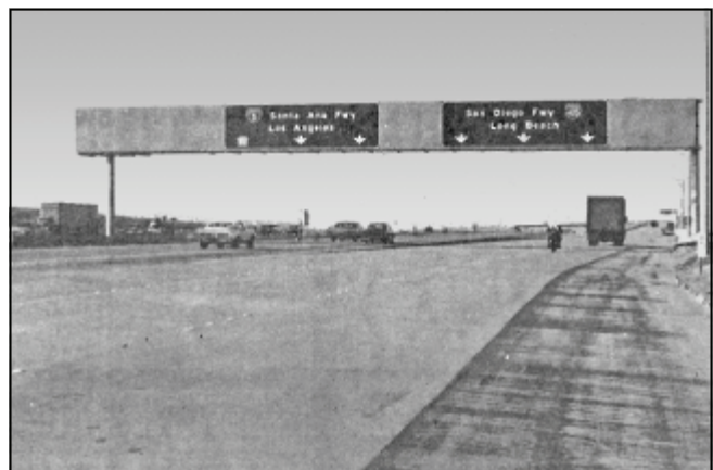
The last segment of the San Diego Freeway opened on January 28 th , giving motorists a direct link to Costa Mesa and other coastal cities as well as the San Fernando Valley.
