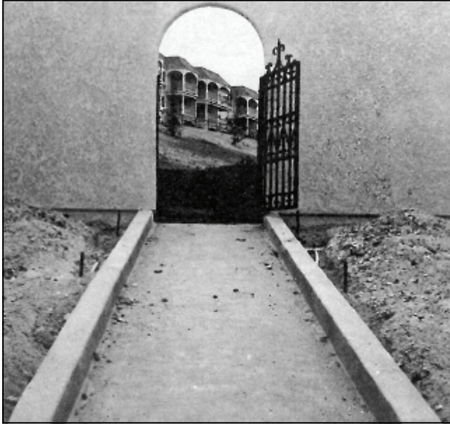
The first four buildings of Phase IV were nearing completion, when this glimpse of a three-story Villa Nueva building was seen through the archway of a Casa Milano on May 1, 1977.
